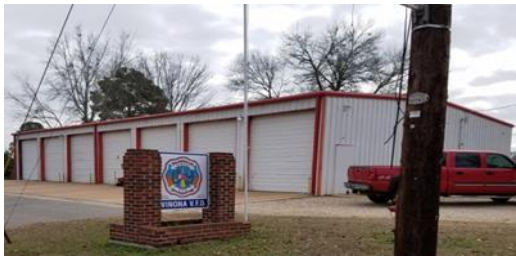
Figure 135: Winona VFD, Station 1
